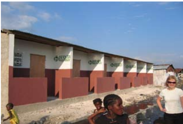
HT trustee, Katherine Coleman inspects the newly constructed houses that Hands Together built for the poor in Cite Soleil.
